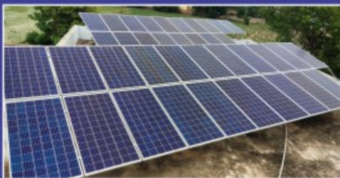
Solar System Setup of 13 kw.
